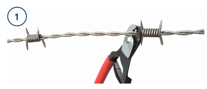
Cut wire at the barb, leaving at least 8 cm I 3 inches of wire to make the join, make sure the end of the wire is tightly wound.
